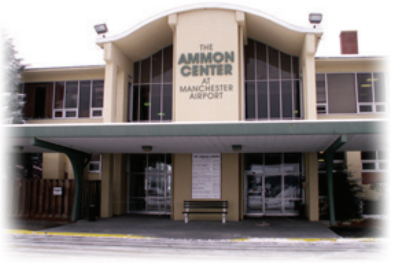
The Ammon Center • Manchester, NH
