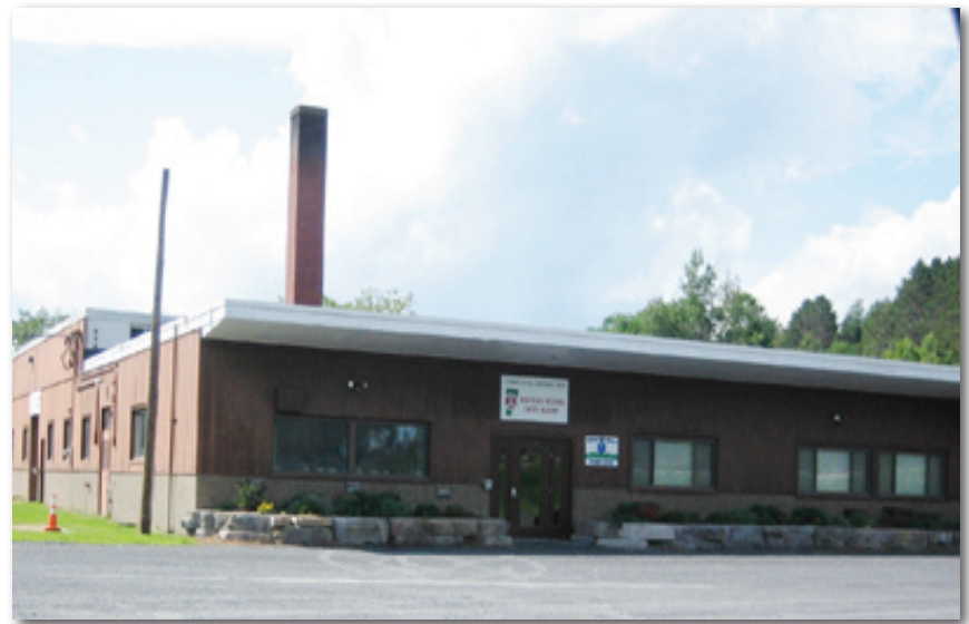
AGC-VT Classroom building • Montpelier, VT
